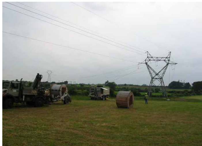
Figure 5.8 Typical Stringing Equipment
