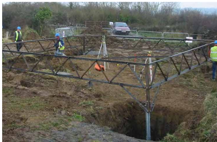
Figure 5.3 Setting Template being prepared for Final Concreting
