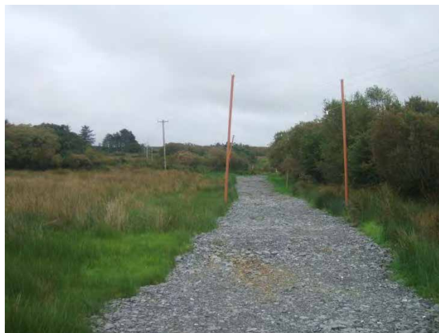
Figure 5.2 Temporary Stone Road
